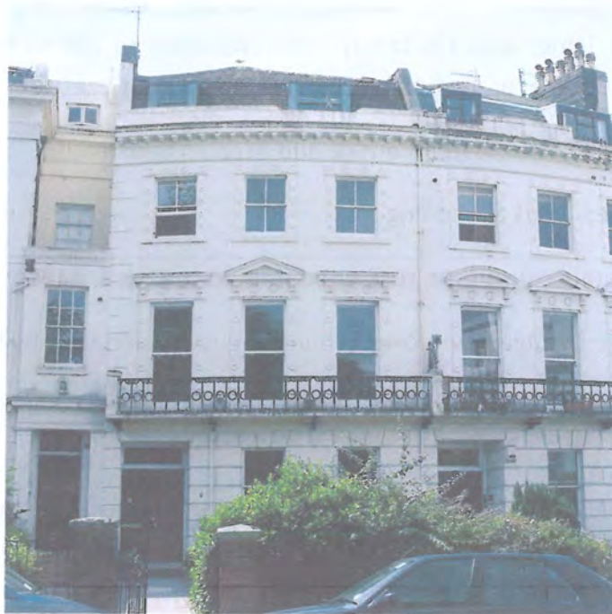
No 6 Montpelier Crescent today.
