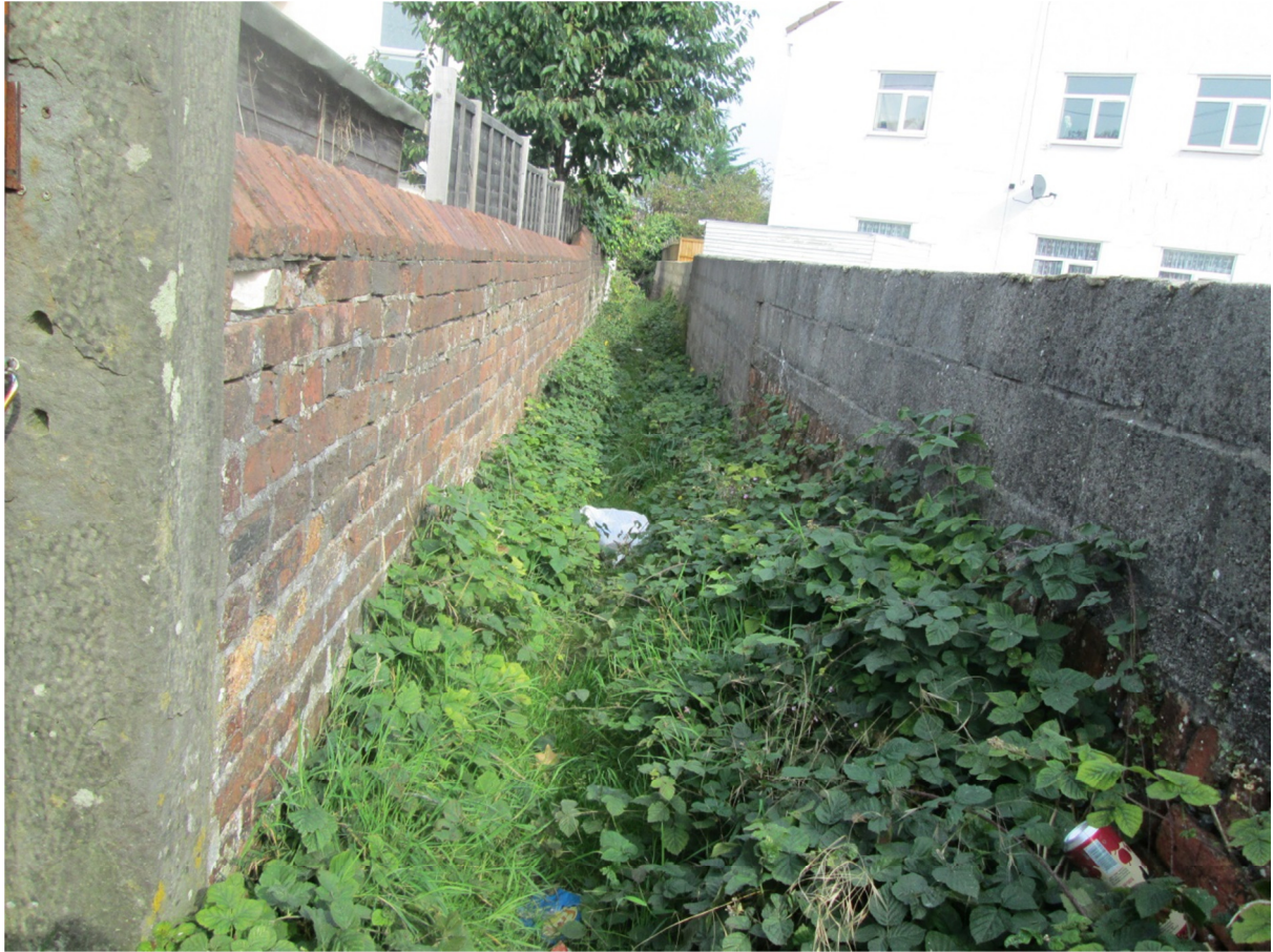
A less congested part of the alley, but still “No through Road”
